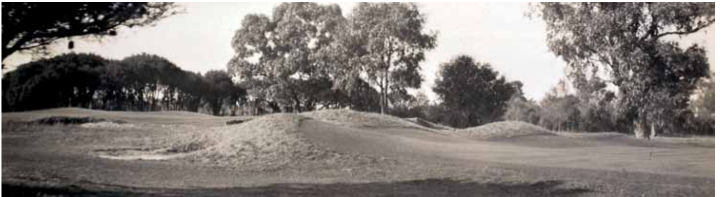
Then (1934) Looking at the 13th and 5th greens from the 14th tee, with the 13th green then raised at the back.
